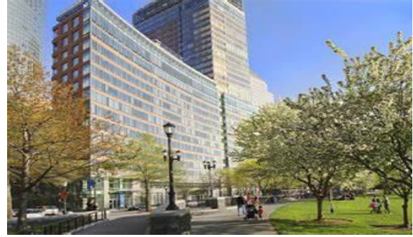
شكل (4) مبنى One River Terrace
