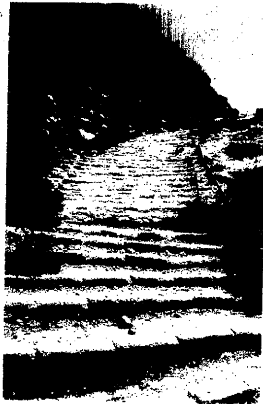
Fig (16): Al-Qala' Stairway-Amman Steps Stones are Taken Away.
