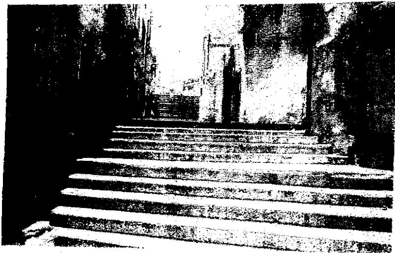
Fig (11): Stairway Route Moving Between Houses and Shops - Jabal Amman
