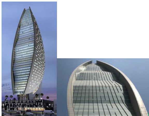
Figure 7 – Iris Bay Tower [40]
