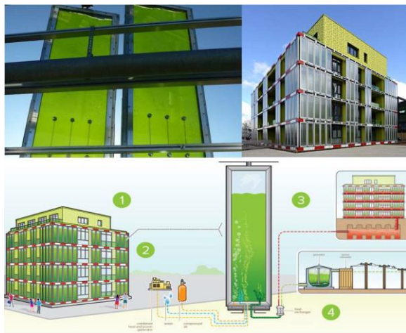
Figure 3 - Bioreactors application facade in Hamburg, Germany [38]
