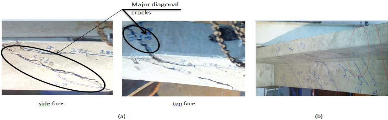
Fig 6: Cracking pattern of: (a) R-C and (b) T-C
