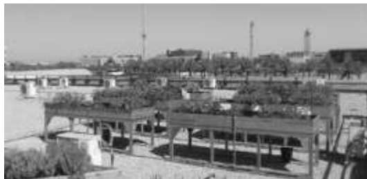
Fig. 3. Faculty housing’s green roof. [16]
